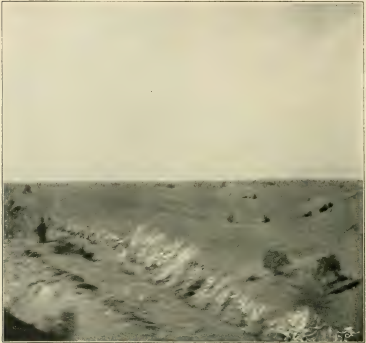
BUNDLES OF FAGOTS USED AS A SAND BARRIER TO PROTECT THE RAILWAY AGAINST THE DRIFTING SAND
